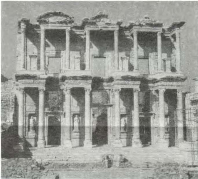
Restored Library at Ephesus (Aegean Tour)
