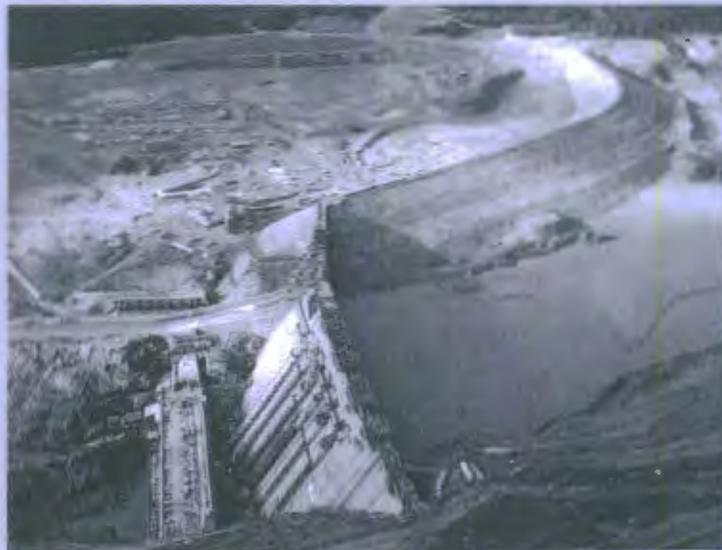
▼ Lock & Dam 26 on the Mississippi exemplifies Dillingham's ability to participate in the biggest projects in the world on a joint venture basis. When finished, 500,000 cubic yards of concrete and 722,000 tons of riprap stone will be placed, and 4.3 million cubic yards of excavation for this 10-year, \$750-million project.
