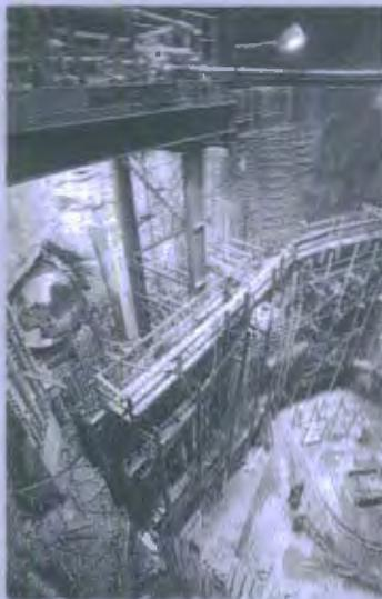
▲ Dillingham built PG&E's 140 MW Kerckhoff Hydroelectric Power Project, including one of the largest silo-type underground powerhouses in the world and a machine-bored 24 foot-diameter by 22,000-foot-long tunnel, all in granite — monumental tasks that would test the mettle of any contractor. Dillingham finished six months ahead of schedule.
