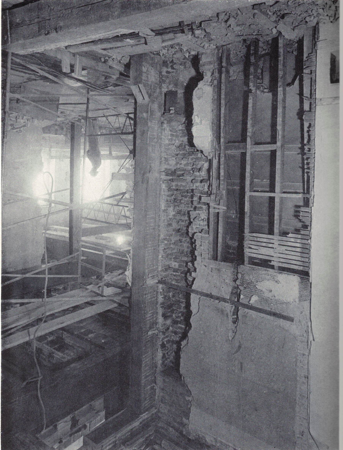
Main Support at Top of Main Stair, Second Floor, under Bearing for T4 Truss
