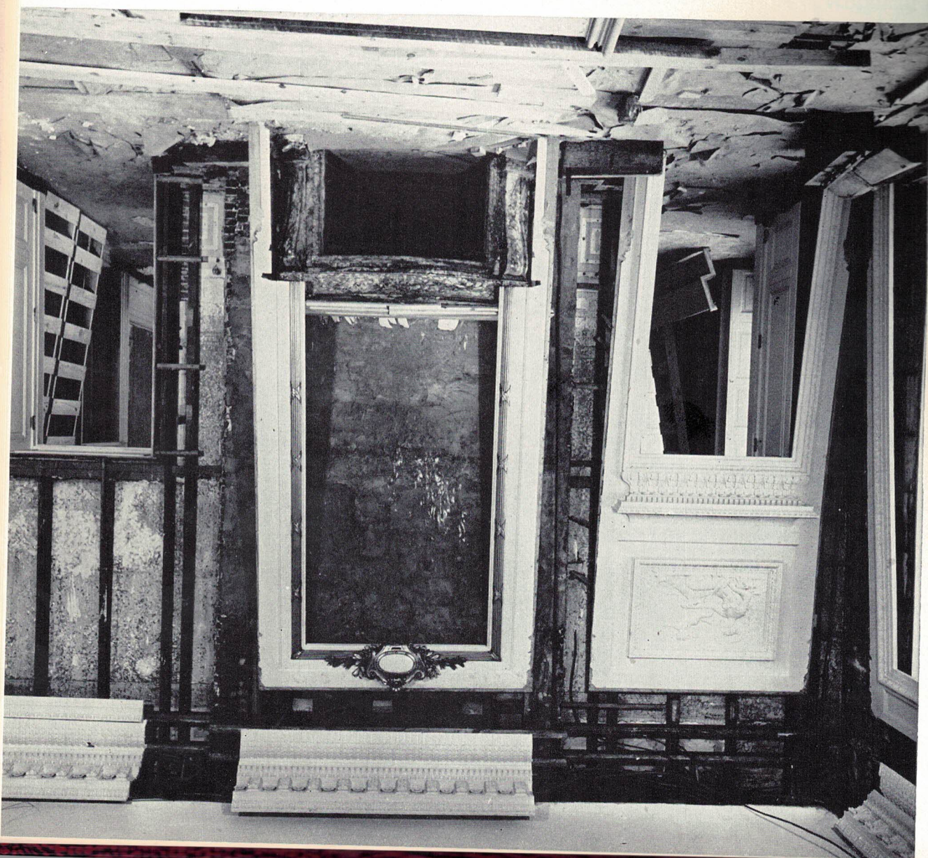
Southwest Corner of East Room Showing Careful Removal of Materials
