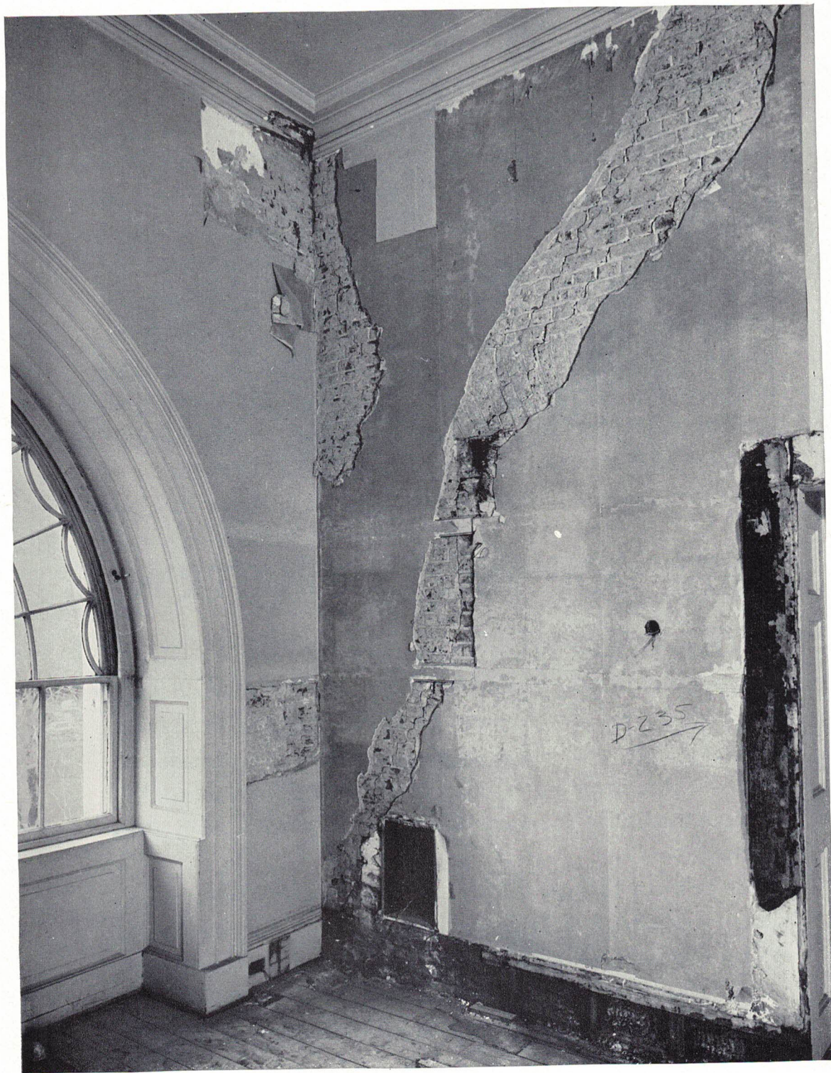
Cracks in the Northwest Corner and in the North Brick Wall in the West Sitting Room, on the Second Floor, as revealed in investigation prior to the Renovation
