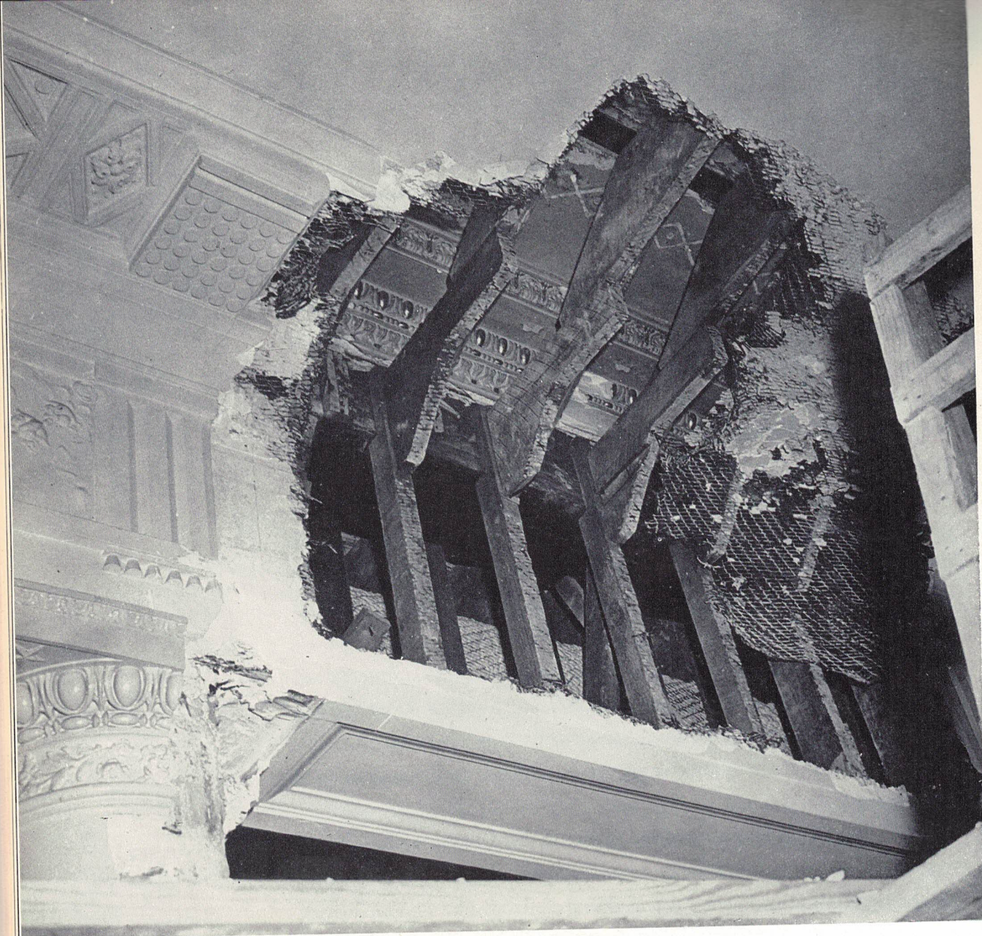
Hoban's Original 1817 Ornamental Plaster Cornice, High-lighted in Gold, in First Floor Centre Hall. Shown Exposed Behind 1902 Plaster Cornice
