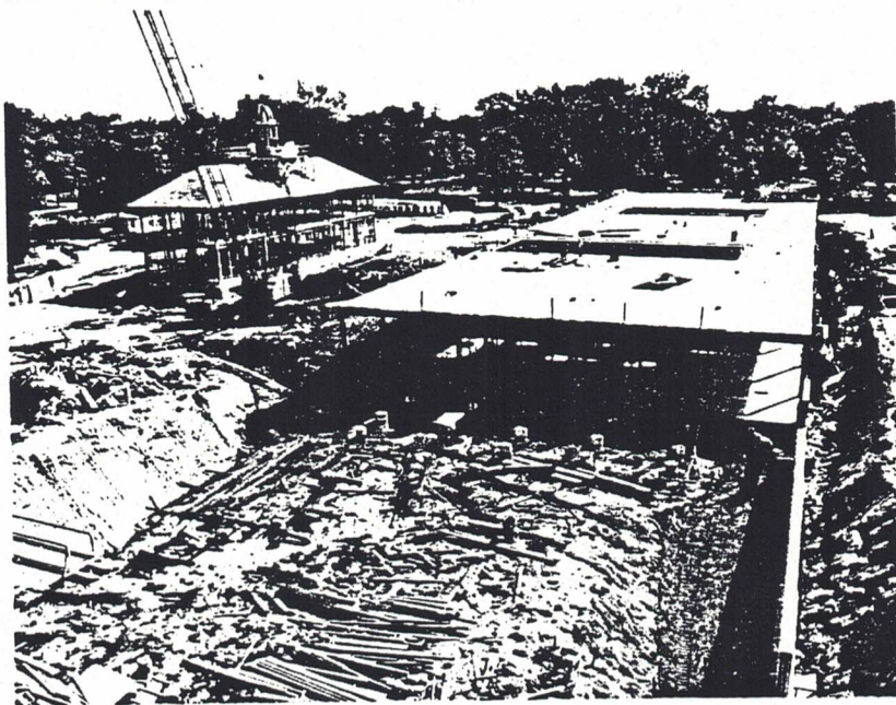
A view of the Gallery and Hospital looking east from S. Henry Street in September, 1983. The rectangular openings in the gallery roof will be covered by filtered glass skylights and indicate the location of two interior garden courts. Initially the west end of the gallery building will be treated as a garden enclosed on three sides by a 12' high brick wall.
