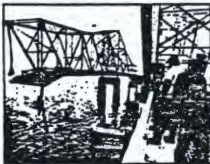
Tampa, Fla., bridge after ship hit support pier in 1980. Deaths were blamed in part on safety flaws.
