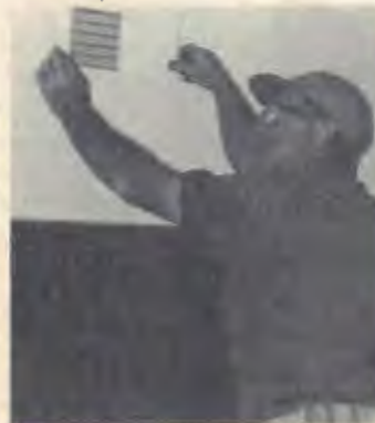
(L-r): Richard Freund, St. Mary Ct. 594, McHenry, Illinois, replacing the heat register in the Oak room; Raymond Smith, adjusting accoustical ceiling tile.
