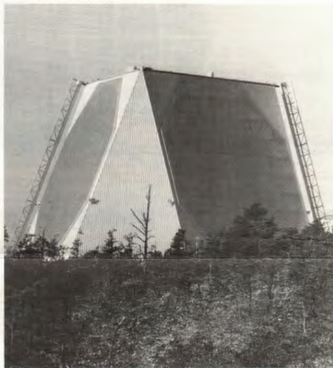
Phased array radar for the PAVE PAWS system. ABM radars are similar in shape but smaller. (U.S. Air Force Photo)
