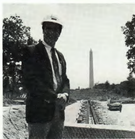
Project Director Robert Doubek making an on-site inspection of construction.
