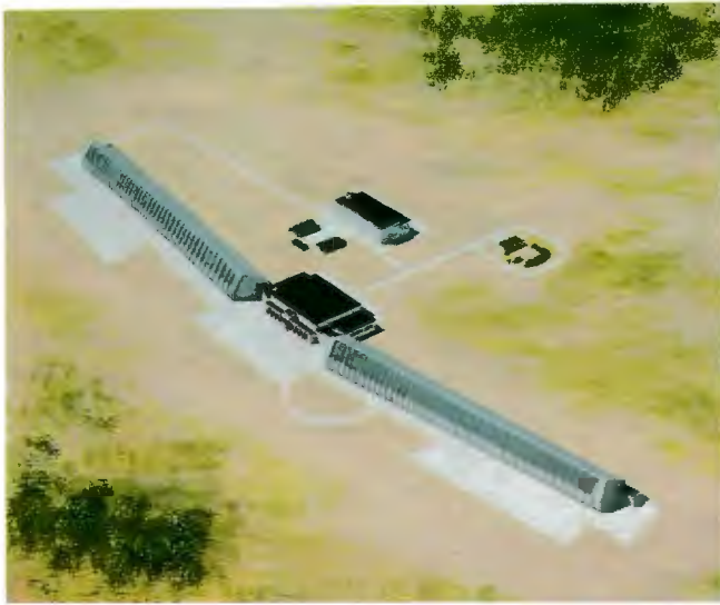
The 11 large HEN HOUSE ballistic missile early warning radars, at left, at six locations on the periphery of the USSR provide warning and target-tracking data in support of the Soviet ABM system. The DOG HOUSE radar, at right, provides battle management for the anti-ballistic missile interceptors around Moscow.
