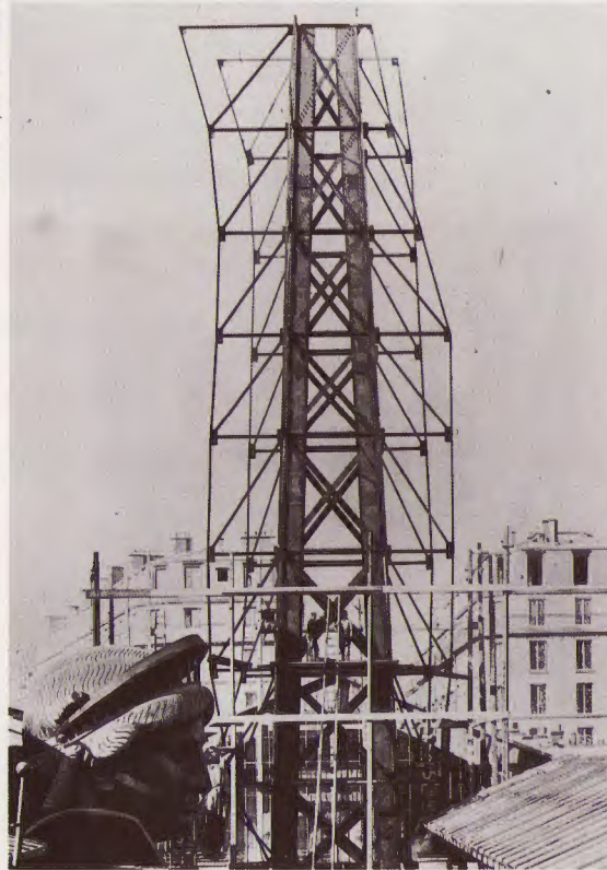
Liberty rose around a central pylon which gave support to the floating curtain.
