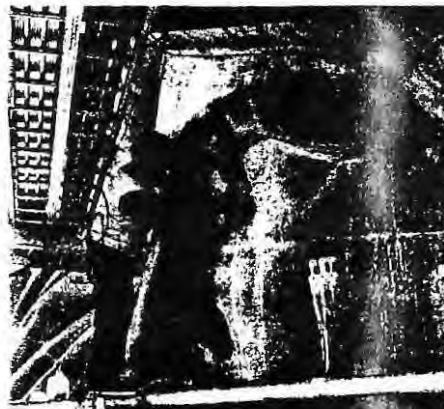
CONSTANCE BASSETT, A PATINIST, STAINS PATCHES NEW COPPER TO MATCH THE REST OF LIBERTY'S FACE
