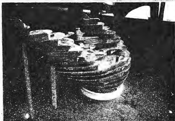
Constructing a small wooden model of the flame was one of the early steps in restoring Liberty's torch to the sculptor Bartholdi's original specifications.
