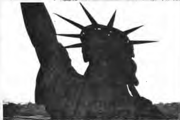
The statue's right shoulder, misaligned by two feet off-center during original construction in Paris, was reinforced, but not corrected.
