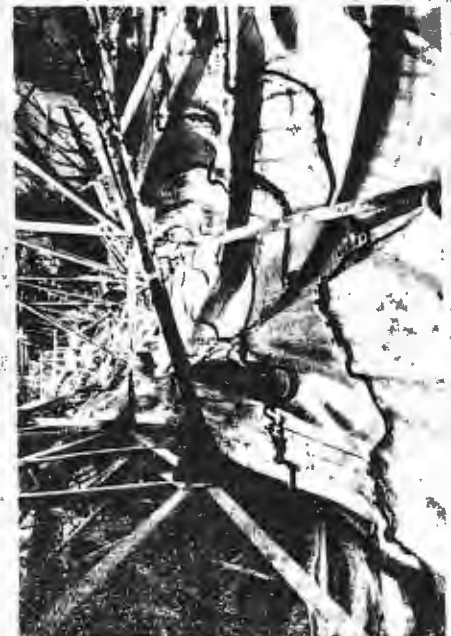
A peek under Liberty's flowing skirts shows the armature-bar supports designed by Alexandre Gustave Eiffel.
